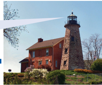
Charlotte-Genesee Lighthouse America's oldest surviving lighthouse on Lake Ontario
